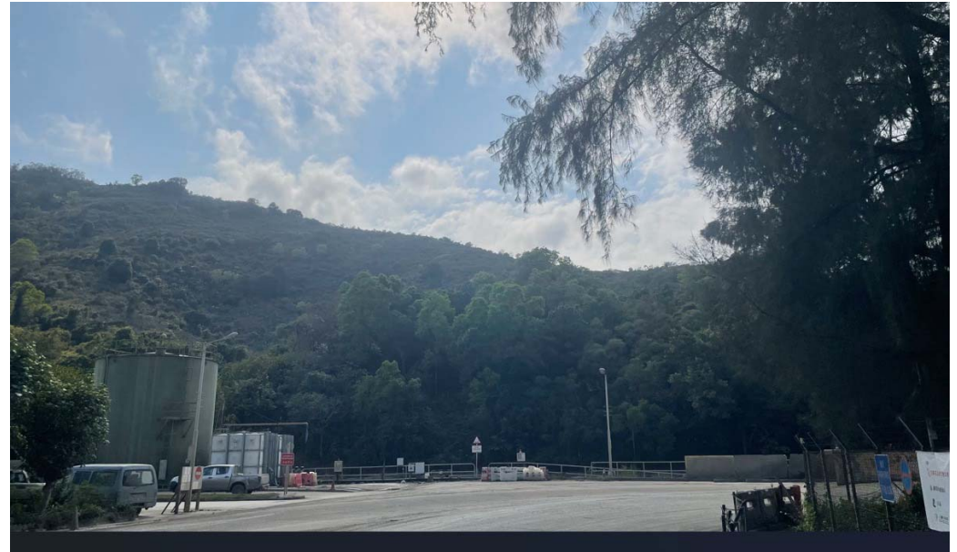
VSR2 - Existing WENT Landfill Site
