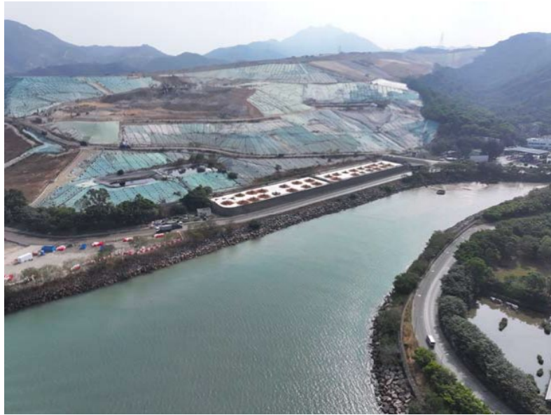
LR10 – Landfill (Construction in Progress)
